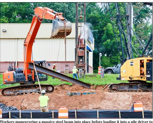
Workers maneuvering a massive steel beam into place before loading it into a pile driver to shore up dirt near the Murphy Highway/515 sinkhole. Photo by Shawn Jarrard
